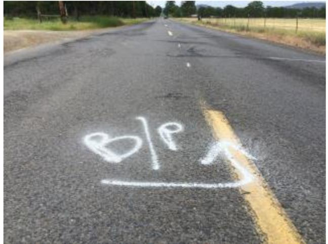
Arrows, and sometimes the use of “B/P”, indicate a blade patch – an area where an asphalt patch is applied over a general area to usually improve ride quality. The new asphalt is spread by use of a motor grader using the blade.
